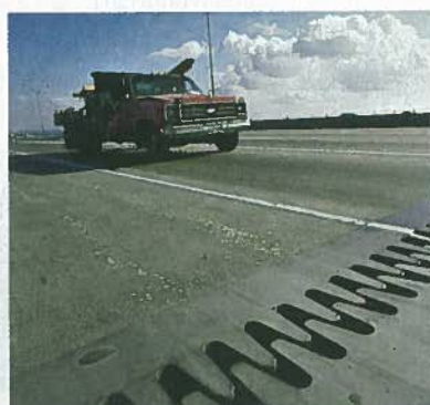
FIGURE 17-3 Expansion joint on a bridge.
